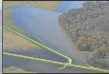
Highway 61 at Low Water Bridge Road
