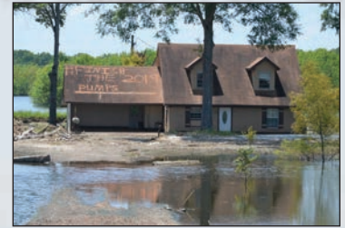
Post flood - Highway 61
