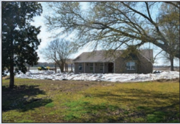
Sandbagged Ring Leveed House
