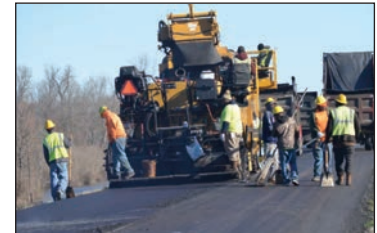
463L - Paving Hwy 465
