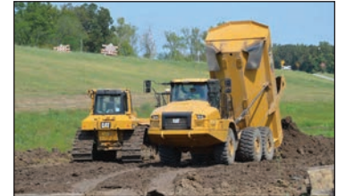
465L - Landside Seepage Berm Construction
