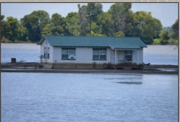
Post flood - Highway 61
