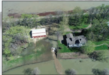
Aerial view of Eagle Lake backwater flooding (3-22-19)
