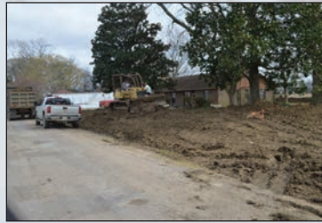
Constructing Ring Levees at Holly Bluff
