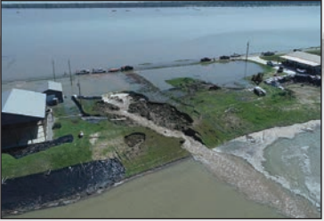
Aerial view of Eagle Lake backwater flooding (3-22-19)
