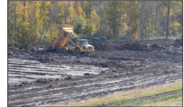
465L - Building Landside Berm
