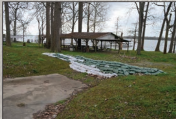
Sandbags at Brunswick Circle Levee & Pennley Road
