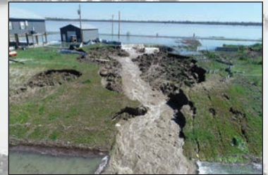
Aerial view of Eagle Lake backwater flooding (3-22-19)
