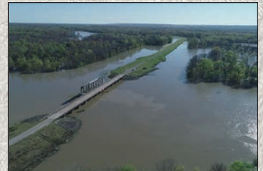
Aerial view of Steele Bayou Structure
