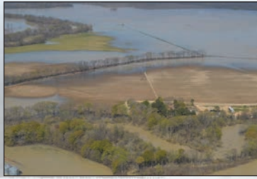
Highway 16 west of Holly Bluff
